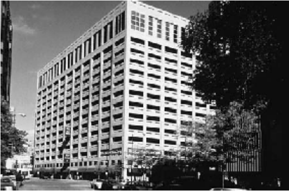
Figure 1.4 Parking structure at 900 N. Michigan Ave, Chicago. High-strength concrete helped to reduce column sizes in this 15-story structure. Courtesy of Portland Cement Association.
