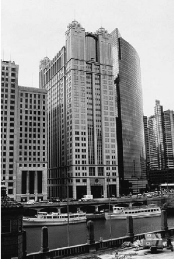
Figure 1.1 Office building at 225 West Wacker Drive, Chicago: constructed with 96 and 117 MPa (14,000 and 17,000 psi) concrete. Courtesy of Portland Cement Association.
