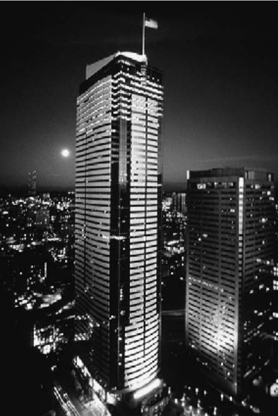
Figure 1.2 Two Union Square, Seattle. Courtesy of Portland Cement Association.
